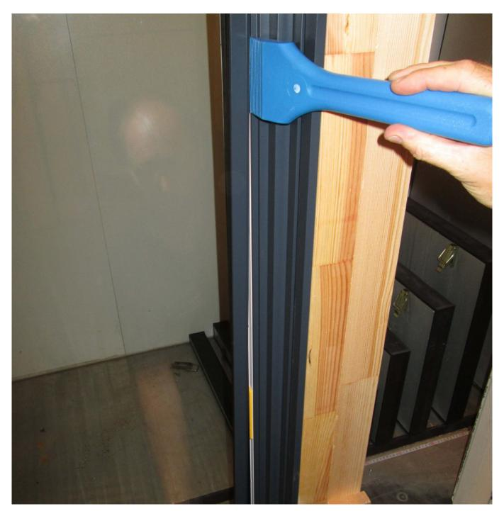
Once the bead has loosened from the jamb, prise off the rest of the bead free using the paddle.
