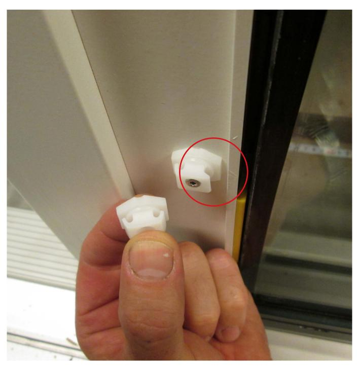
Any damaged clips should be replaced before the aluminum glazing beads are refitted. Pay attention to white stripes on the clips, this may mean that they have been bent, making it difficult to fit the beads again.
