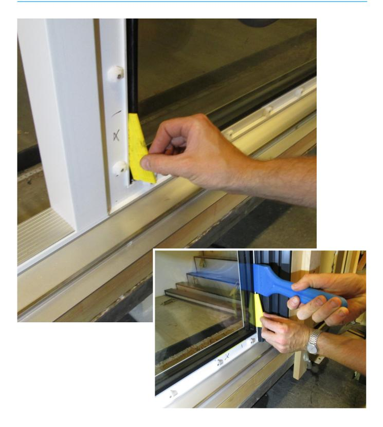
Insert the remaining setting blocks. Setting blocks positioned according to the marks that were made during the removal, and drawing PRO-500-063 on page 21
