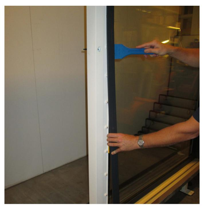
Once the bead has released its grip from the first clips, prise off the rest of the bead free using the paddle.
