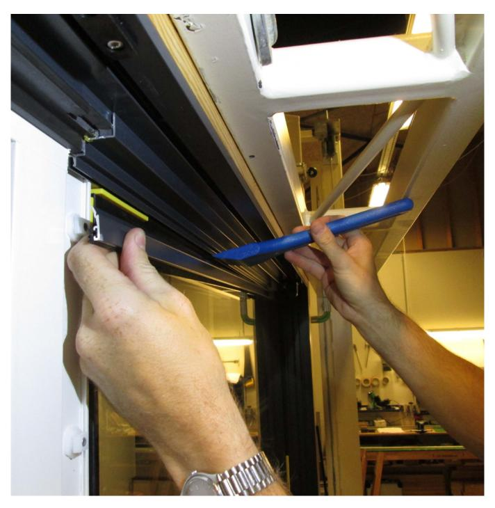
Once the bead has loosened from the frame, prise off the rest of the bead free using the paddle.
