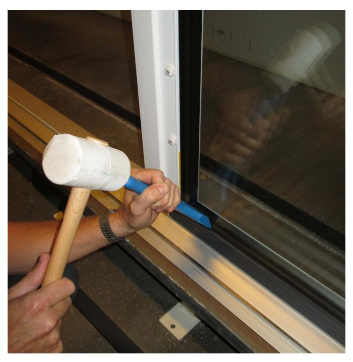
The glazing bead on the bottom cill is loosened by tapping the paddle carefully in between the glazing and the bead.
