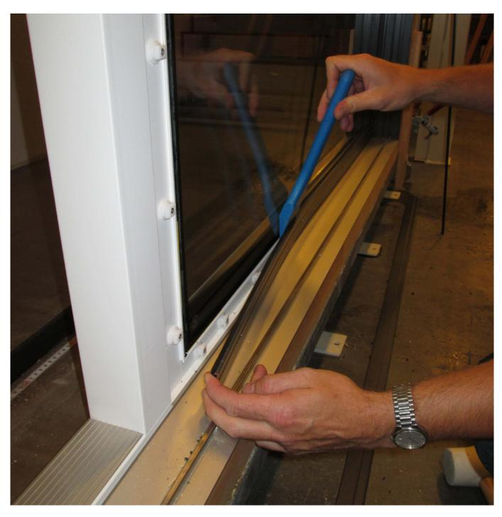
Once the glazing bead has released its grip from the first clips, prise off the rest of the bead free using the paddle. Again, be aware of any damaged clips.
