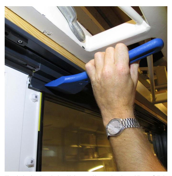
The glazing bead on the head is loosened by tapping the paddle carefully in between the bead and the aluminum frame.
