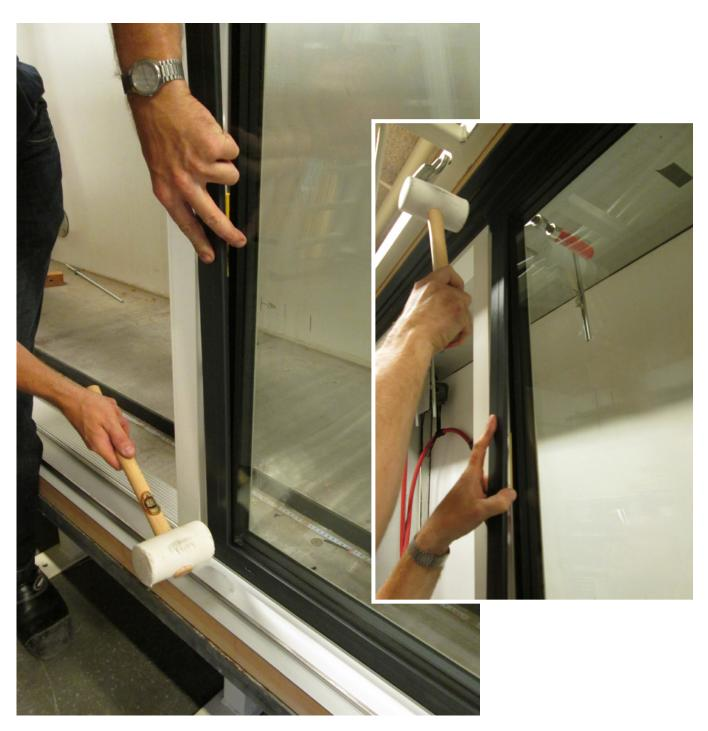
When the head and cill glazing beads are fitted, both sides can be mounted. The procedure for the glazing bead at the mullion is: Tap the bead carefully onto the clips, first at the bottom and then the top.
