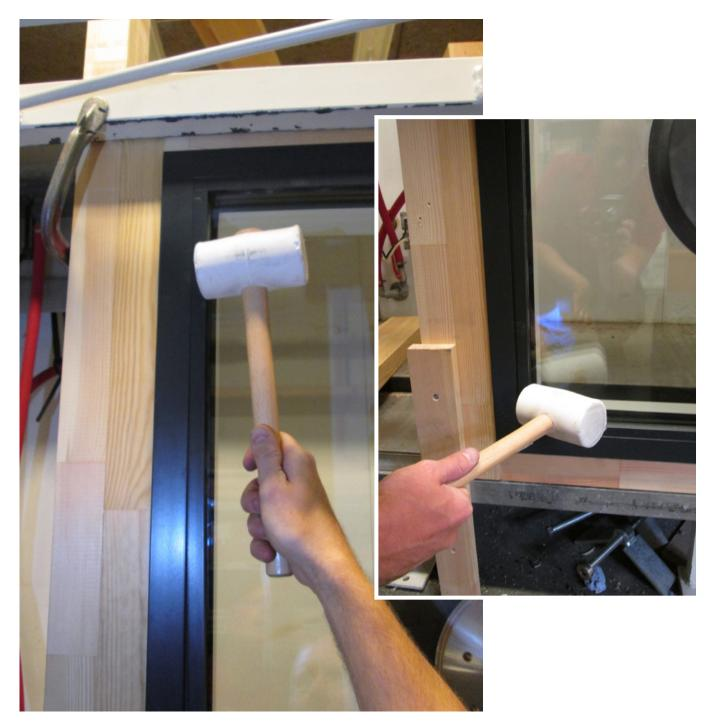
The glazing beads are fitted by carefully tapping them into place with a rubber hammer. The beads are fitted ends first. Start with the head bead, then the cill and at last both jambs.
