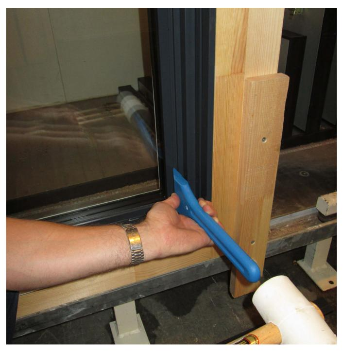
The glazing bead on the jamb is loosened by tapping the paddle carefully in between the bead and the aluminum frame.
