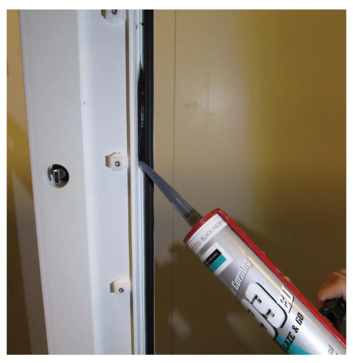
Apply new sealant to the frame before inserting the new glazing, positioned according to existing sealant / setting blocks.
