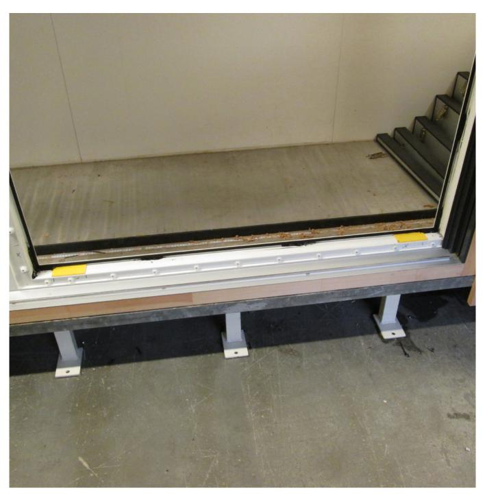
Lay setting blocks in the bottom first. Setting blocks positioned according to the marks that were made during the removal, and drawing PRO-500-063 on page 21
