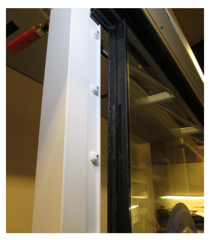
The glazing can now be removed from the frame.
