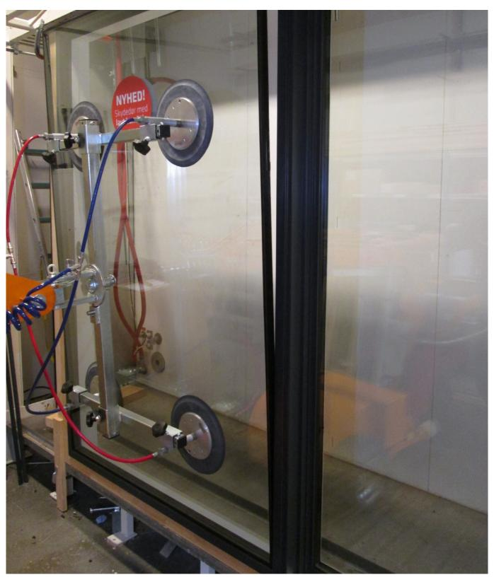
The new glazing can now be inserted. Insert bottom first, and tilt the top into place.
