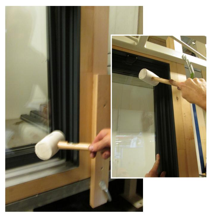
At the opposite side of the mullion i.e the jamb, use same method as at the head. The glazing bead is fitted by tapping it carefully in place with a rubber hammer, first at the bottom, then the top.
