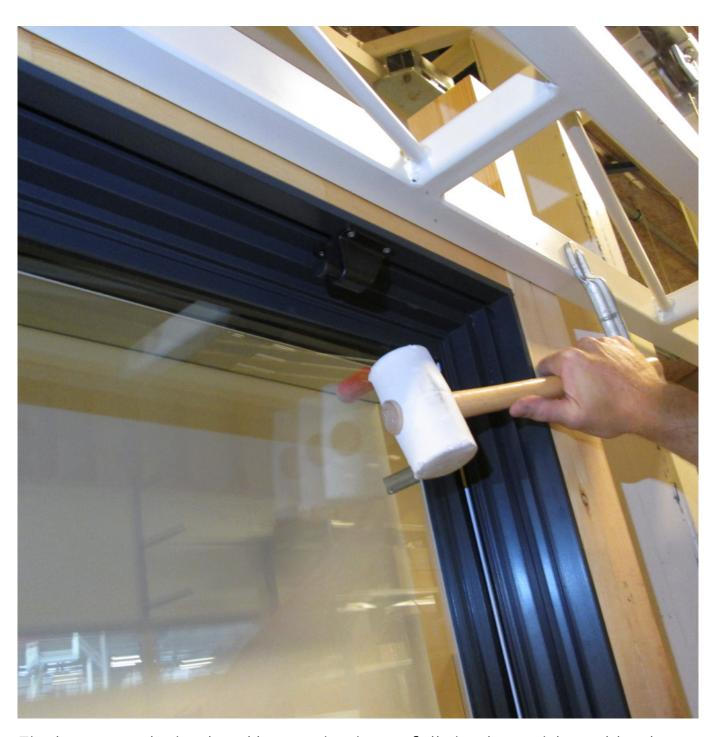
Fit the upper glazing bead by tapping it carefully in place with a rubber hammer.
