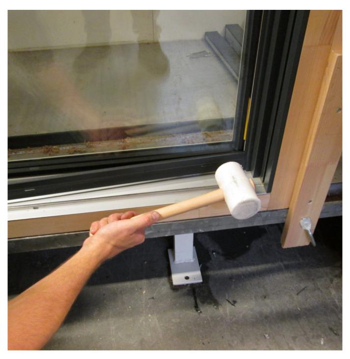
Then fit the bottom glazing bead. This is done by tapping the bead carefully onto the clips.
