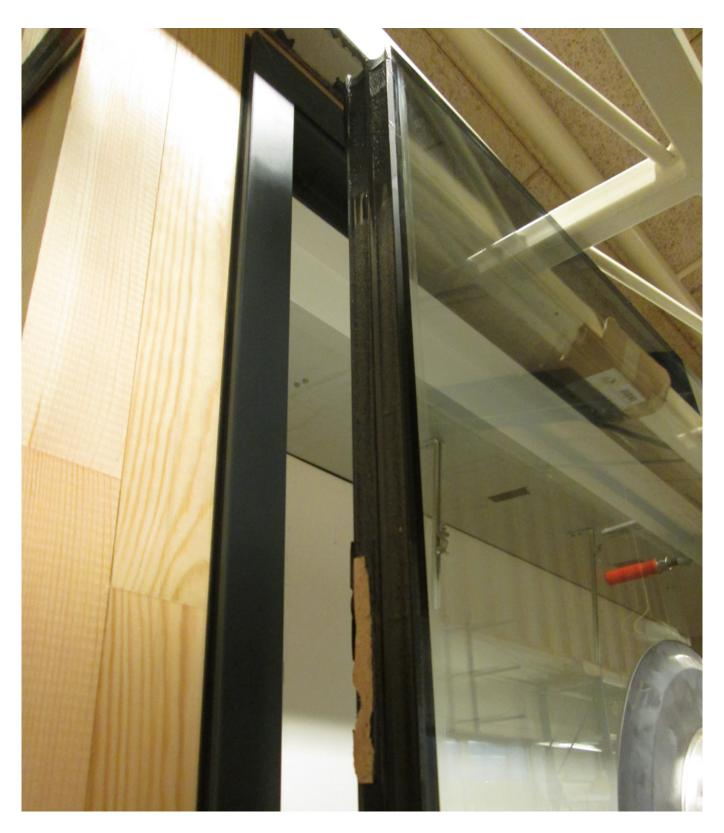
The glazing can now be removed from the sash, by tilting from the top.
