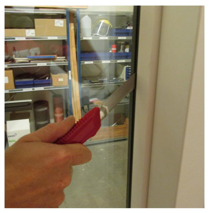
To loosen the glass, cut along the inside of the door too.
