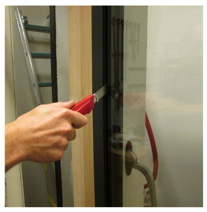
The glazing is cut free of the sealant with a long sharp knife.
