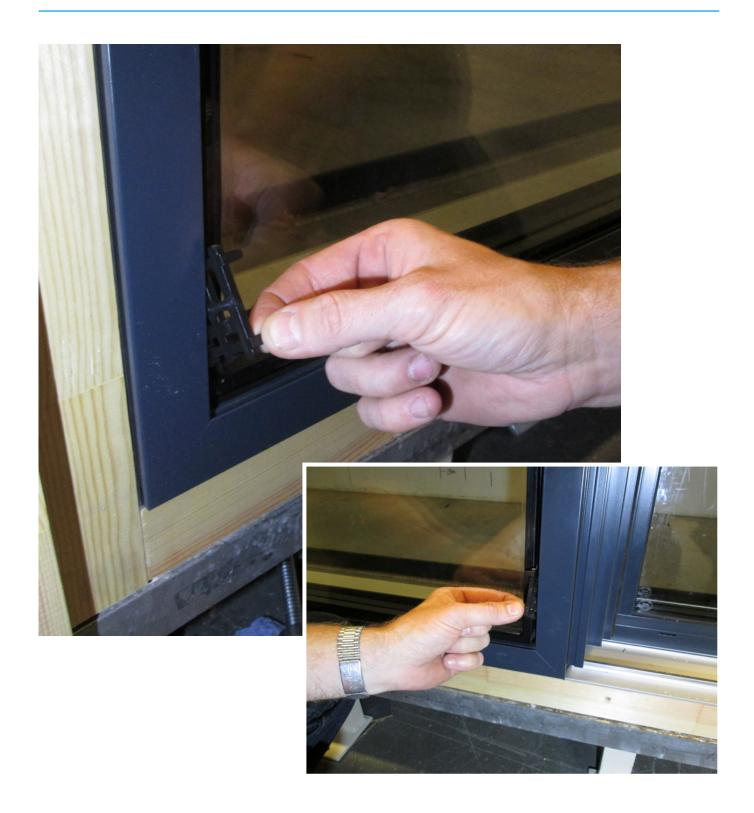
Insert the remaining setting blocks. Setting blocks positioned according to the marks that were made during the removal, and drawing Pro-500-063 on page 38
