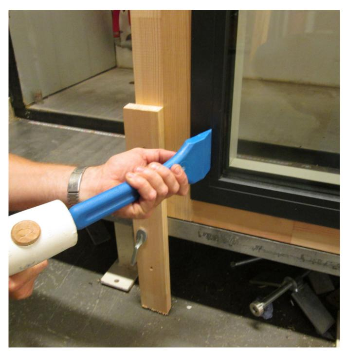
In the sliding part, all glazing beads are dismounted a like. Begin with the aluminum glazing beads in the sides, then bottom and top.
